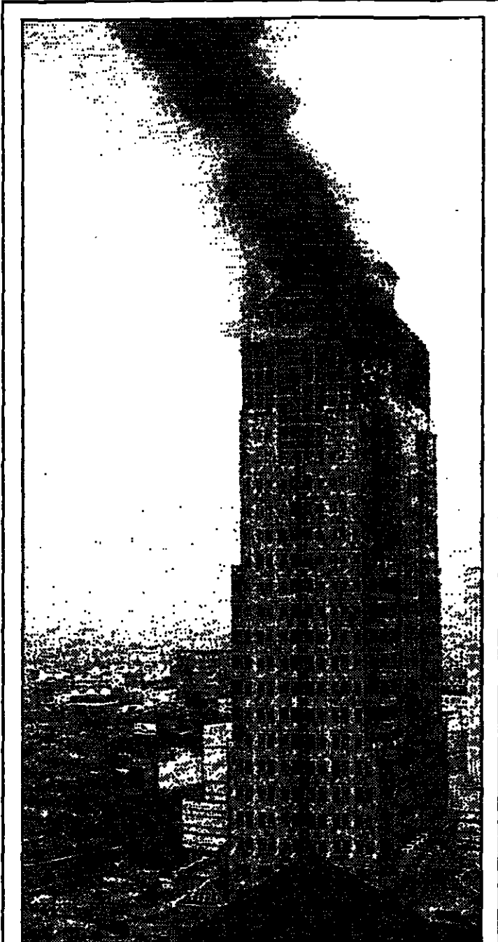
Up in smoke A newly constructed 35-story tower, part of Indonesia's central bank, billows with smoke in Jakarta yesterday. The cause of the blaze was not immediately known. (AP)
